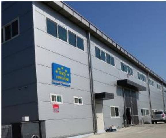
▲ Head Office and Factory 1
